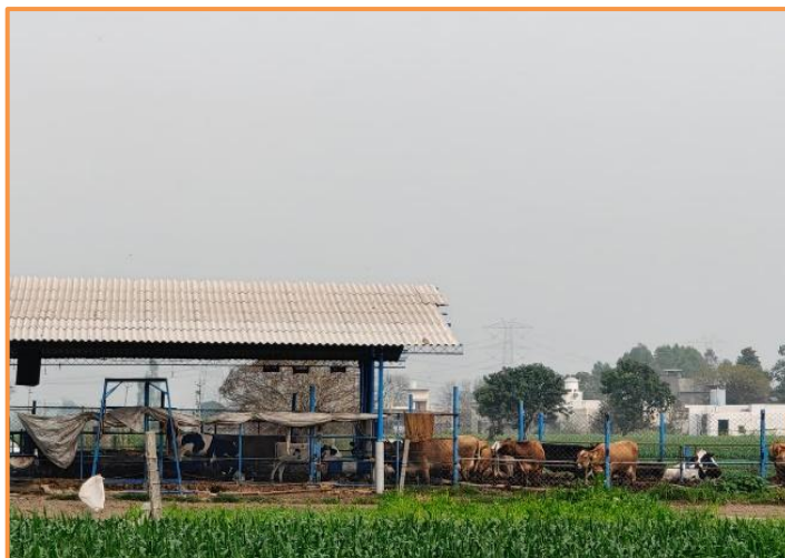
Fig2: Dairy Farm Infrastructure
