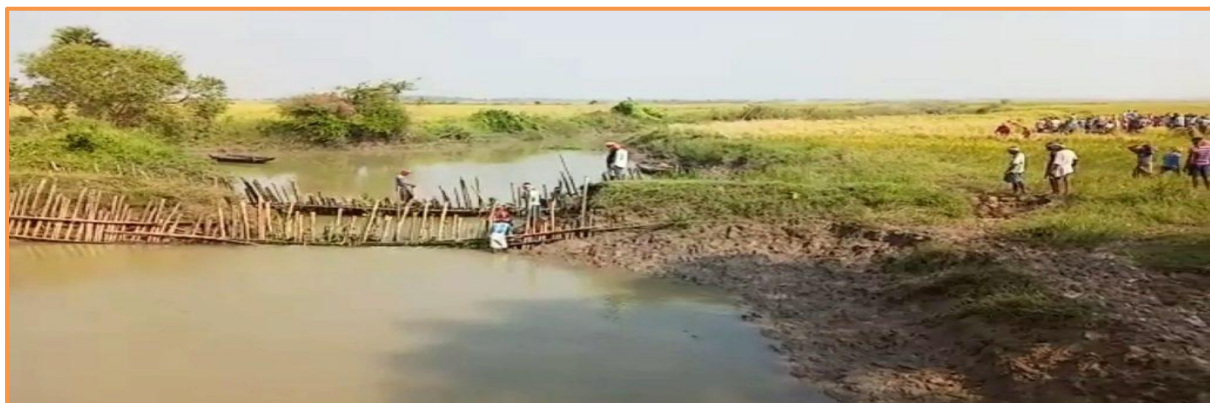
Figure 1: Farmers Building a Check Dam in Gajapati, 2024 (Description: Farmers construct a check dam in a Gajapati village, conserving rainwater.) (Source: WOTR, 202)
