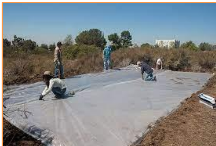
Fig 2. Application of polyethylene sheets to soil (Source)
